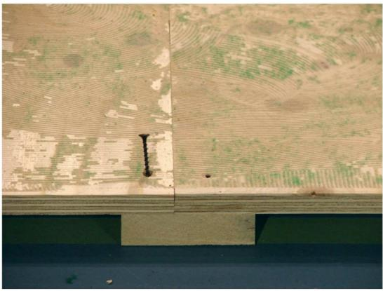
2. Add a **strong border** around the field. Note that the robots may weigh as much as 40 kg, and reach velocities of up to four meters per second, which corresponds to a kinetic energy of 320 Joule. Although robots crashing into the field border will be penalized with a red card,
