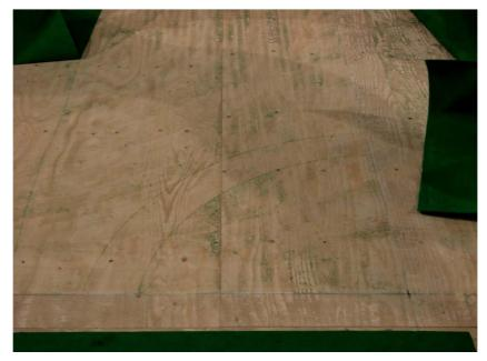
4. Glue green carpet to the wooden floor at areas of the field that are not covered by white lines, and glue white strips of carpet to the floor where the lines should be.
